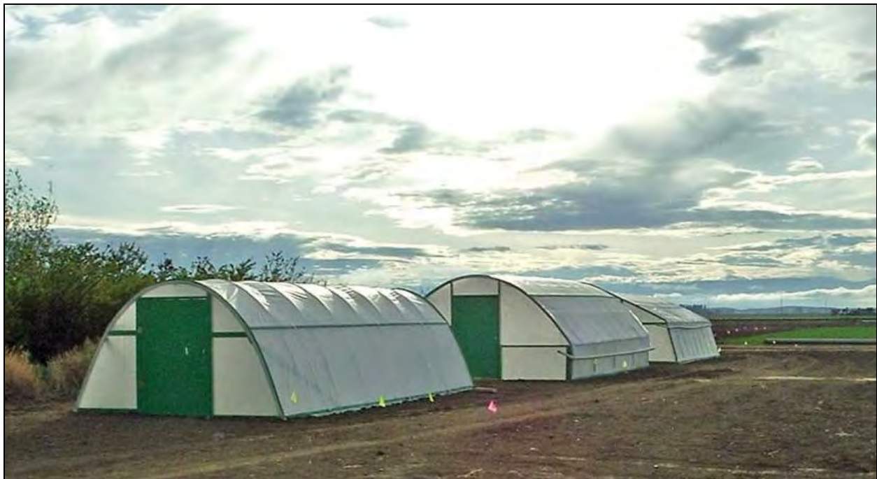
Figure 1.1. Three styles of high tunnels: straight hoop, hard sided, and gothic at the Powell Research and Extension Center. (Photo: Sandra Frost)
