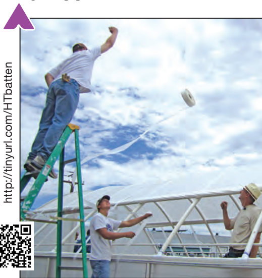
Figure 40. Throwing batten tape over structure for attachment between ribs.
