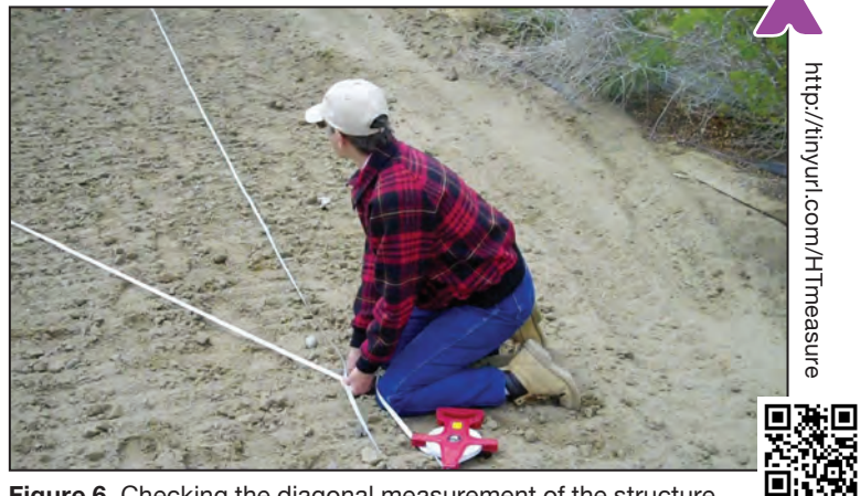
Figure 6. Checking the diagonal measurement of the structure.
