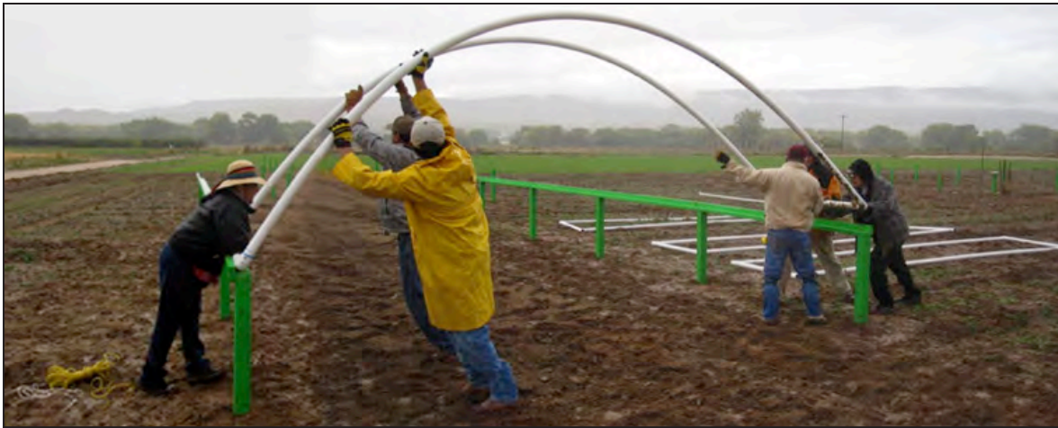
Figure 14. Method used to position rib assembly onto wooden base.
