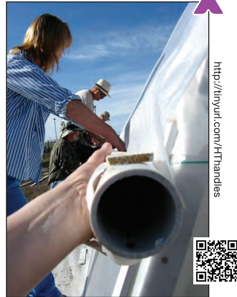
Figure 39. Attaching lath strips to rollup side handle.
