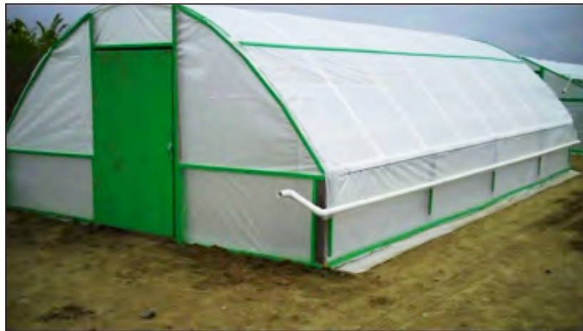
Figure 1. Completed 16' X 32' Hard-sided high tunnel.
