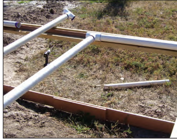
Figure 20. Scab over butt joint of base plate.
