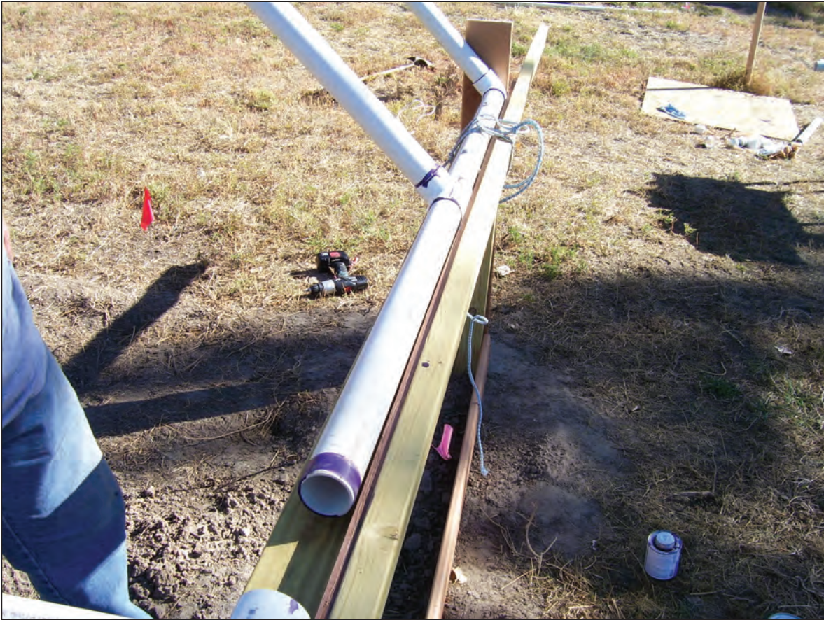
Figure 16. Spacer cleaned/primed and cemented into “T” joint of the first rib assembly.
