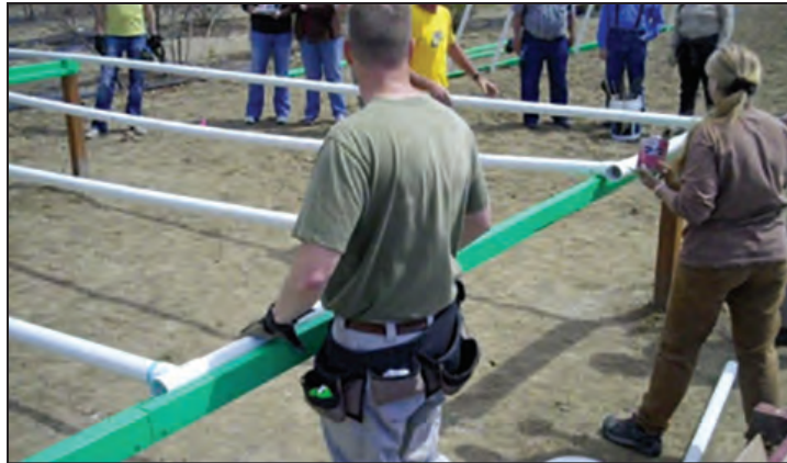
Figure 12. Rib assembly placement prior to attachment to top rail.
