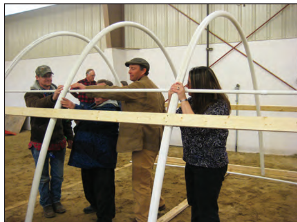
Figure 29. Structural (wooden) and irrigation purlins.
