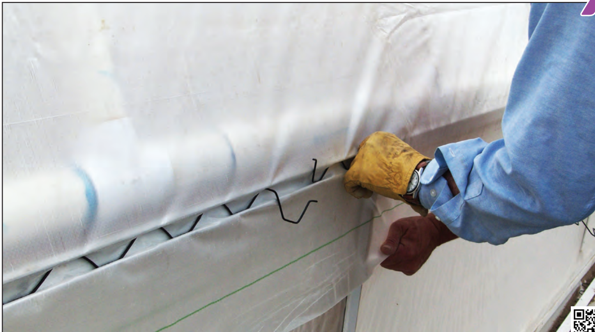
Figure 38. Holding the poly skin in the wiggle wire channel with wiggle wire.
