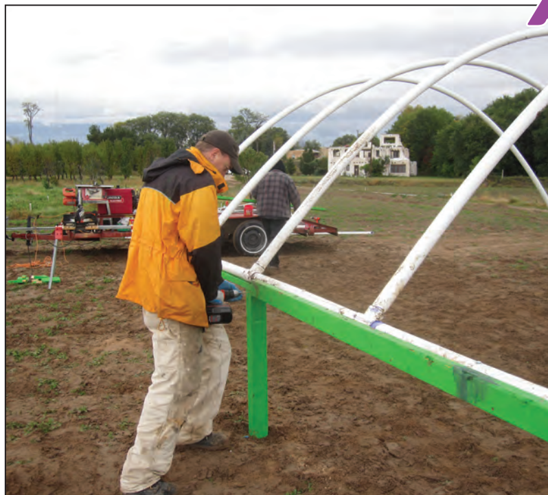
Figure 19. Removing the temporary side rail.
