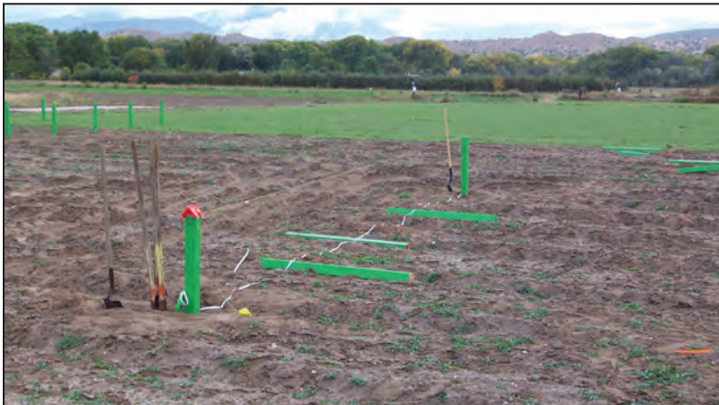
Figure 7. Establishing the Corner Posts.
