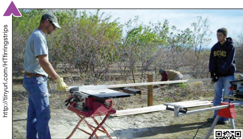
Figure 2. Ripping lath material.
