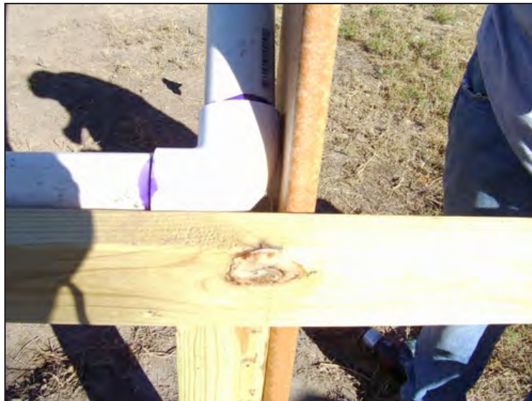
Figure 13. Temporary plate on end of structure to keep first rib assembly flush.
