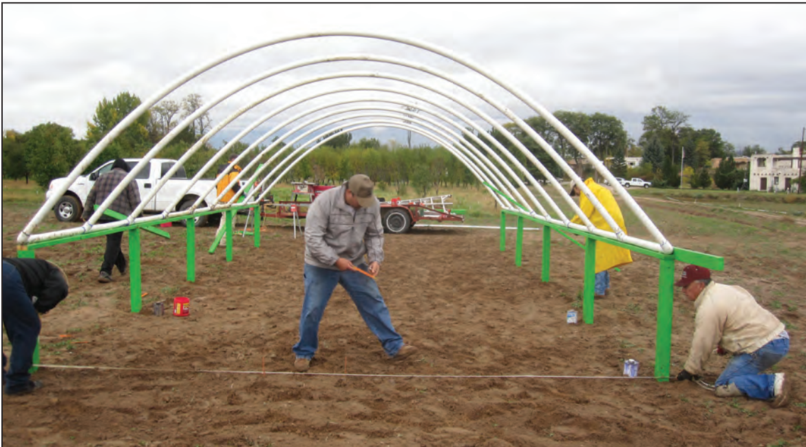
Figure 21. Establishing end wall layout.
