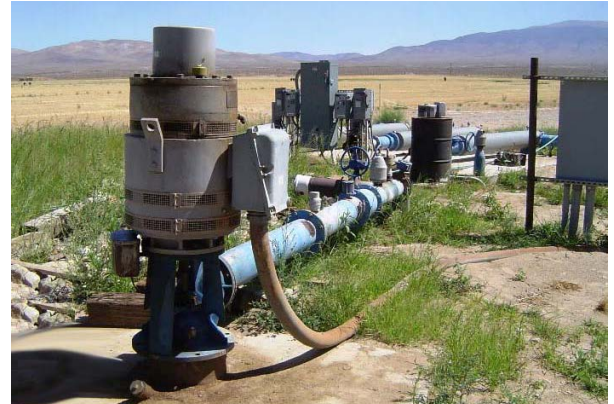
Evaluating your pumping plant can help to identify efficiency issues and areas that can be improved, possibly identifying money saving improvements.
