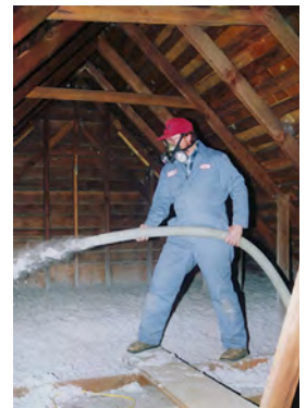
(Photo Community Services Consortium, NREL 17430 http://images.nrel.gov/viewphoto.php?imageld=6318114 )
