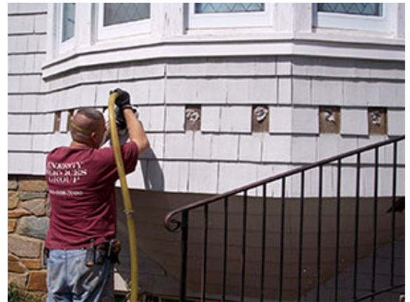
Existing above ground sidewalls are most commonly insulated by removing siding or drilling holes into the sidewall and blowing loose-fill into cavities.
