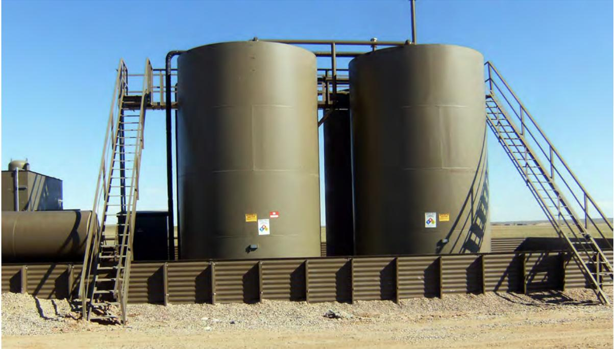
**Figure 12.** Metal berms are easier to maintain and more cost effective in the long term.
