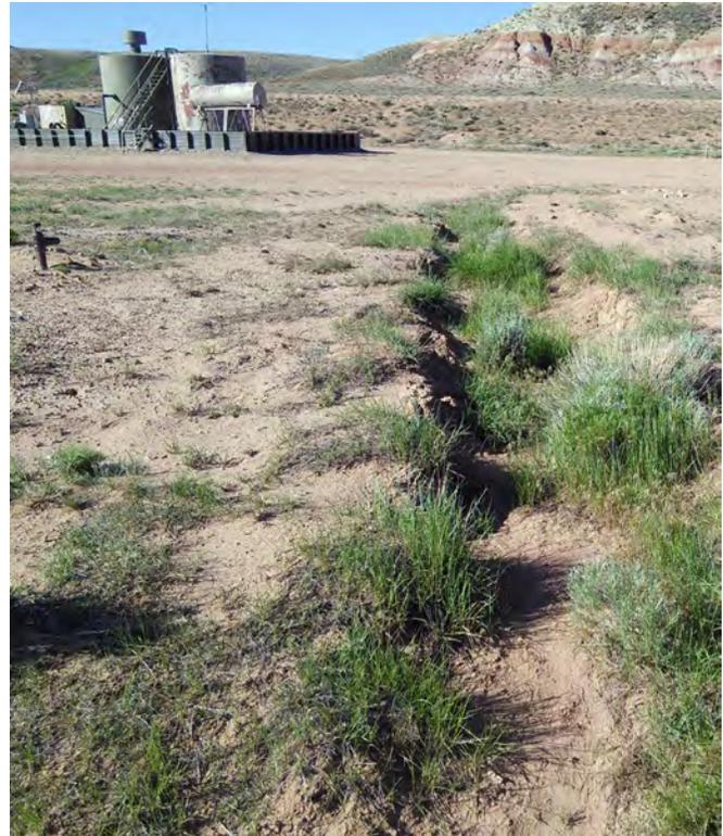
**Figure 6.** Subsidence can be avoided by compacting fill during site recontouring prior to application of topsoil. Once interim reclamation is in place, sites should be monitored for signs of subsidence that require further maintenance.
