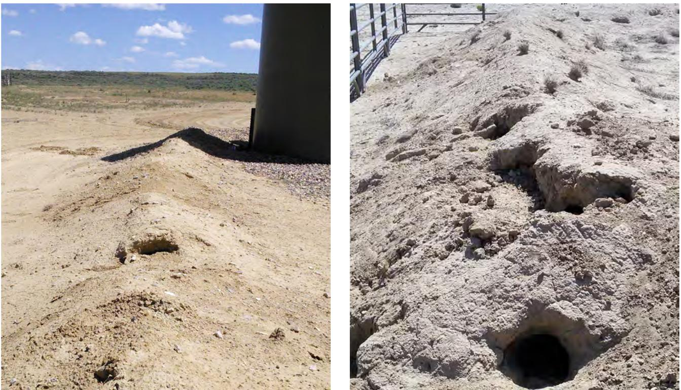
**Figure 11.** Earthwork berms are easily damaged by wildlife or other activities at a well site, and greatly increase the risk of berm failure in case of a spill, which can contaminate interim reclamation.
