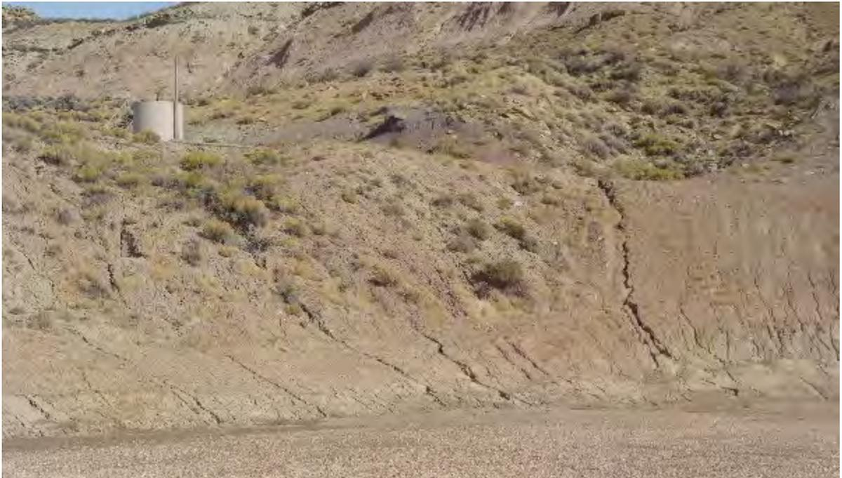
**Figure 2.** Ineffective recontouring can result in steep slopes and poor site stability.
