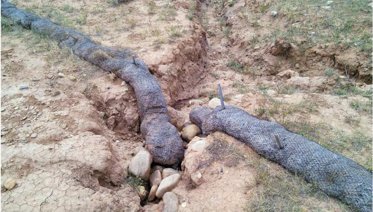
**Figure 5.** Failure of straw wattle, leading to rill and gully erosion. Proper installation is necessary to avoid failure. In this case, wattles may not be sufficient to prevent erosion and other measures are needed.
