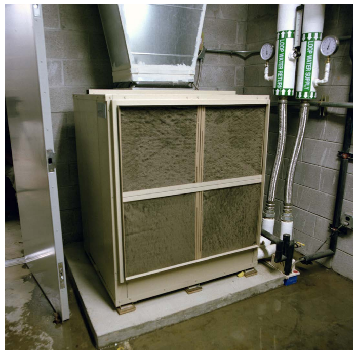
Geothermal heat pump Photo by Craig Miller Productions, NREL O2400 http://images.nrel.gov/viewphoto.php?imageld=6315656
