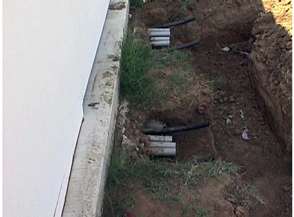
GSHP Loop field entering a building Photo: Robert R. Jones ,NREL 07094 http://images.nrel.gov/viewphoto.php?imageId=6313766
