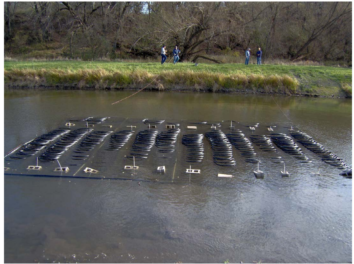
Pond Loop Being Sunk Photo by Mark Johnson (Marktj at English Wikipedia) - Own work. Licensed under Public Domain via Commons - https://commons.wikimedia.org/wiki/File:Pond_Loop_Being_Sunk.jpg#/media/File:Pond_Loop_Being_Sunk.jpg
