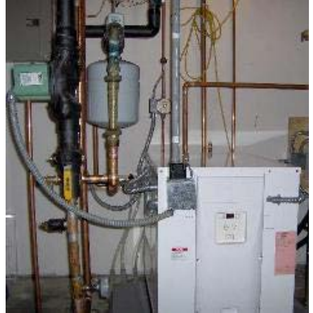
Water to Water Heat Pump
