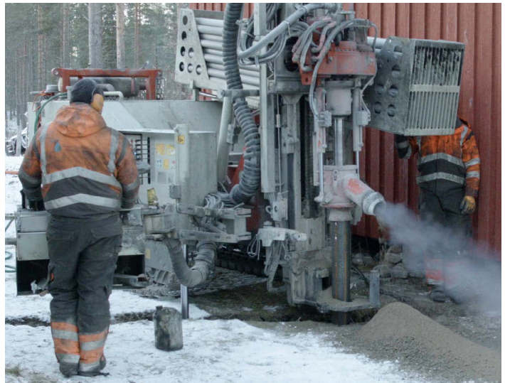
Geothermal drilling for residential heating Photo by Olli Niemitalo - Own work. Licensed under CCO via Commons https://commons.wikimedia.org/wiki/File:Geothermal_drilling_for_residential_heating.jpg
