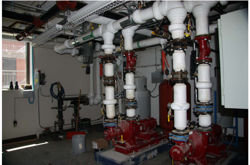
Ground source heat pump system
