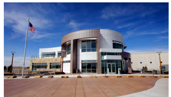
The NCAR-Wyoming Supercomputing Center in Cheyenne, Wyoming. Photo: University of Wyoming
