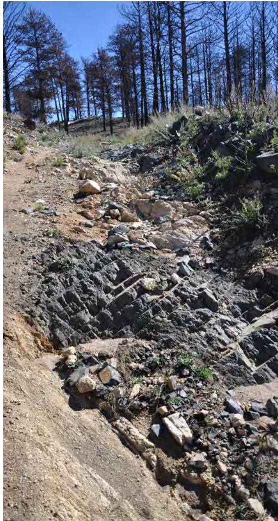
Figure 3. Fires such as the 2012 Arapaho can result in increased runoff and soil erosion during rainfall events, especially during unusually wet periods. That was the case shortly after the fire burned across RRS and surrounding lands in the north Laramie Mountains, when more than 2 inches (5+ centimeters) of precipitation fell during a significant rainstorm in July. (Photo by S. Williams)
