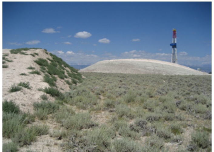
Segregated topsoil (left) and underlying materials (right) near natural gas drilling pads on the Jonah Field.
