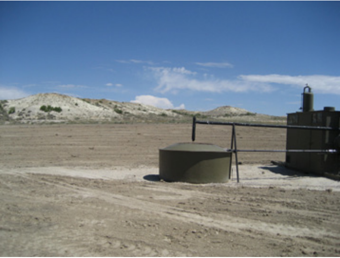
Topsoil has been respread, packed, and seeded on a natural gas drilling pad near Wamsutter.
