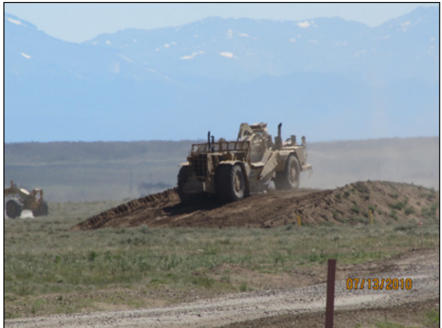
Respreading topsoil
