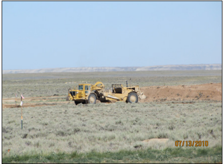
Stripping topsoil
