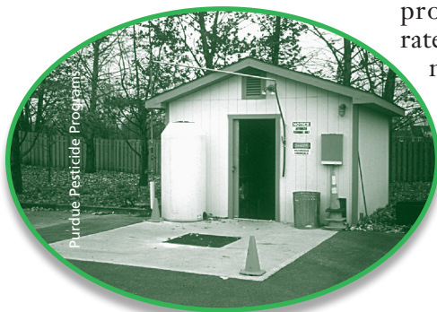
Maintain a well designed, secure pesticide storage facility with highly visible warning signs. Keep it well ventilated and located where water damage is not likely to occur.
