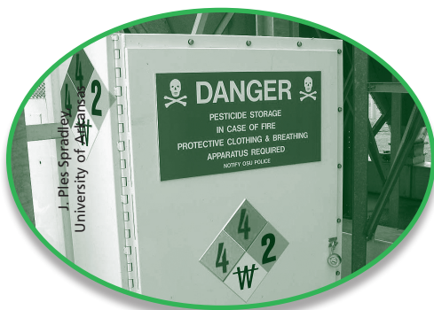
A National Fire Protection Association (NFPA) warning on a storage box for fumigants. The strikeover on the letter W in the white diamond alerts firefighters not to use water to put out a fire.
