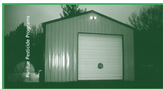
Outside lights on a pesticide storage building help prevent theft and vandalism.
