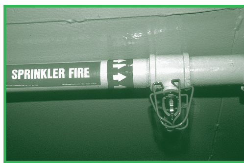
Install fire detection systems such as this sprinkler system with a sensor.
