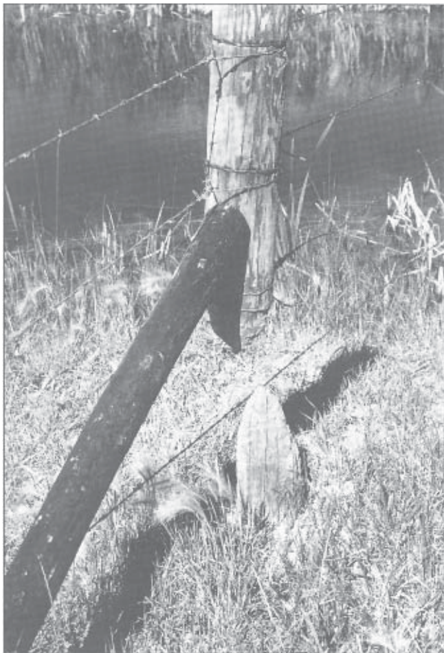
Figure 11. Obvious beaver damage of a unique form (Photo by Rich Olsen).
