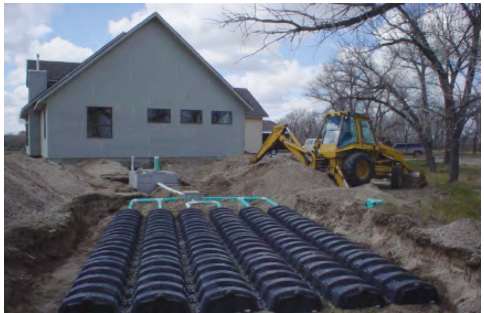
Conventional gravity fed septic system with concrete tank and distribution box. Drainfield is a bed configuration with graveless chambers.
