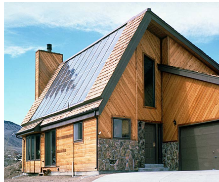
This house in Golden, Colorado uses flat plate water heating panels Photo by Warren Getz, NREL 00655 http://images.nrel.gov/viewphoto.php?imageld=6308655
