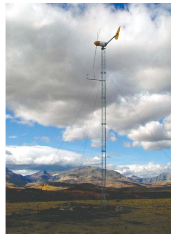
Latticed tower. Photo by Doug Nelson, NREL 14675 http://images.nrel.gov/viewphoto.php?imageId=6327128
