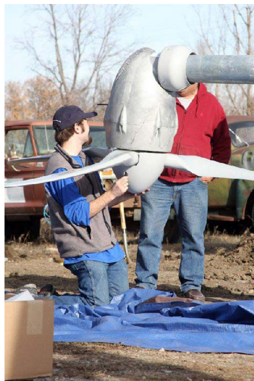
Crew attaching blade to a turbine at the Elkhorn Valley School in Nebraska Photo by Judi Sigler, NREL 16254 http://images.nrel.gov/viewphoto.php?imageId=6326109
