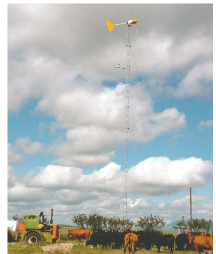
10 kW Bergy Wind Turbine in Stanford, Montana. Photo by Jessica Raker, NREL 14677 http://images.nrel.gov/viewphoto.php?imageId=6327130
