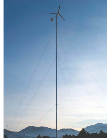
Guyed tilt-up monopole tower Photo by Mark Harris, NREL 16742 http://images.nrel.gov/viewphoto.php?imageId=6326130
