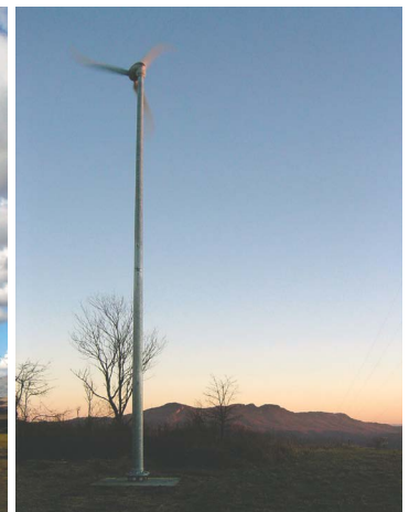
Monopole tower. Photo by Appalachian State University, NREL 15303 http://images.nrel.gov/viewphoto.php?imageId=6326045
