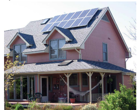
Photo by Namaste Solar Electric NREL, 15620
