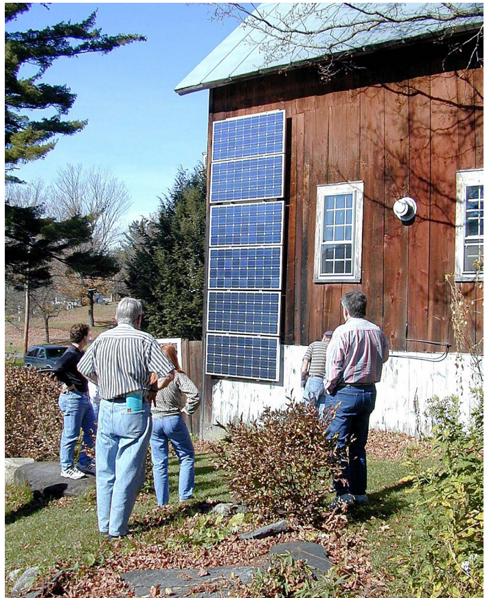
In an area prone to power outages, one homeowner in Strafford, Vermont, installed a set of batteries and attached a PV panel to the side of his barn to keep them charged. Photo courtesy of Alan Ford / NREL:09499
