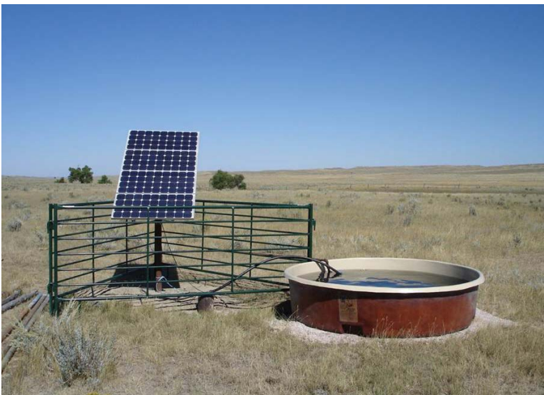
Solar Livestock Watering System Photo courtesy of Steve Fletcher, University of Wyoming. CC BY-NC 3.0 http://farmenergymedia.extension.org/
