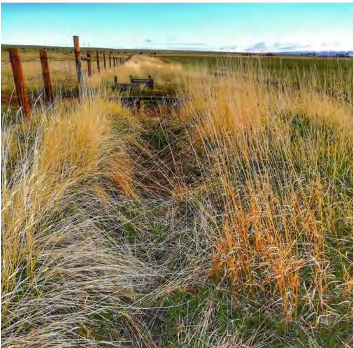
Figure 1. Irrigation ditches can become overgrown with vegetation and plant litter that can physically slow the rate of flow of irrigation water, clog gates and grates and harbor weeds, insects and disease. Long-term lack of maintenance can also render these unusable.
