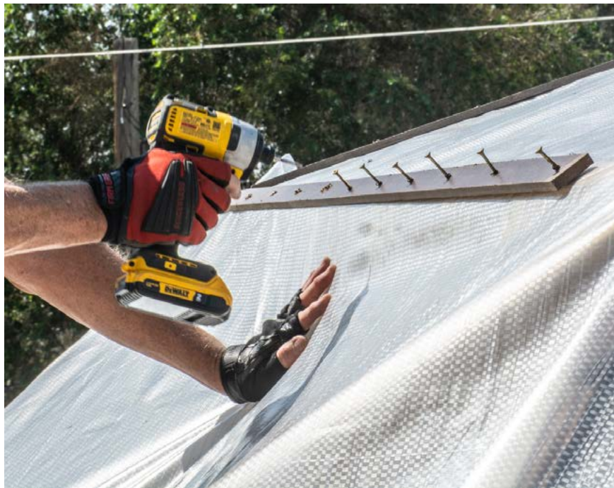
Attaching the skin with prepped lath.
