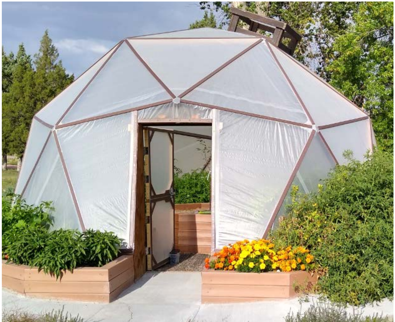
Figure 1. 22-ft 2V geodesic dome constructed in Fort Laramie, Wyoming, in 2021. Photo: Jeff Edwards
