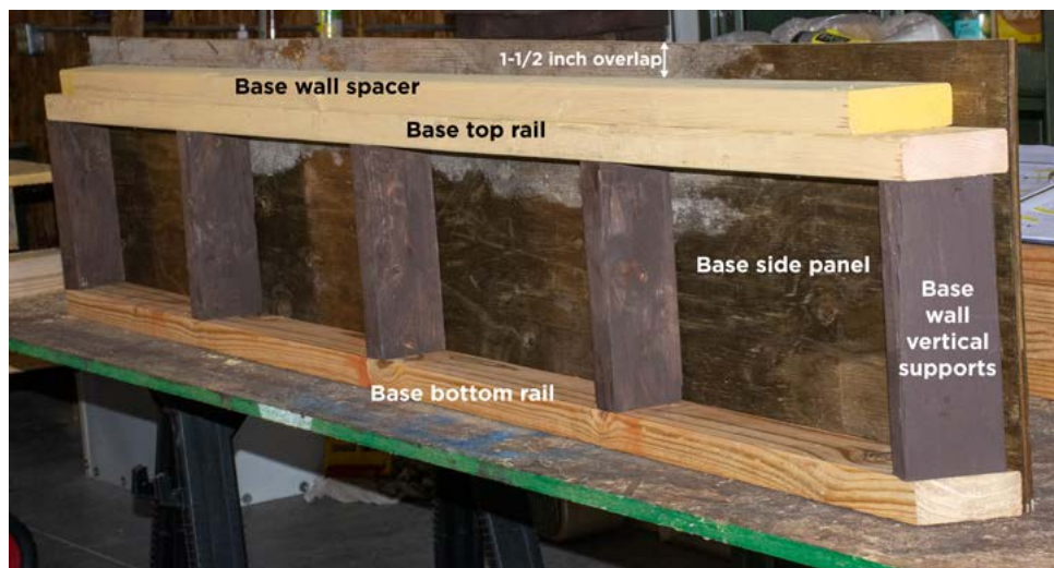
Figure 3. One assembled base wall section. The plywood side (base side panel) is on the exterior of the geodesic dome. The image represents the base wall when building the dome without raised beds
